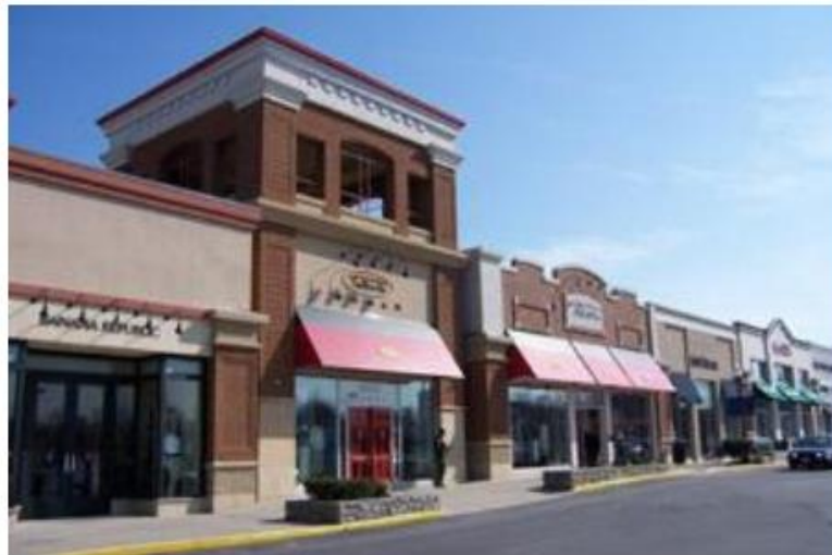
Figure 3: Illustration of façade treatments such as pilasters, projections, and material changes to provide a visual façade offset.
