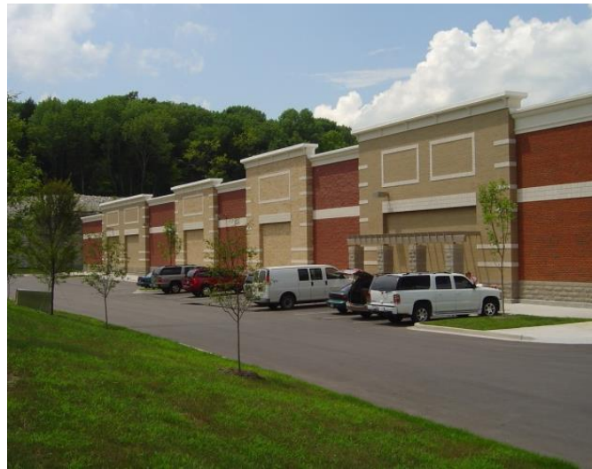
Figure 2: This figure shows two methods of using architectural features to create wall surface relief on wall elevations that are not the primary elevation.
