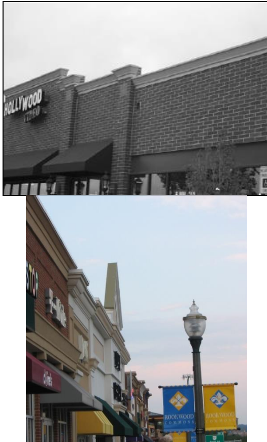
Figure 5: Parapet walls with cornice treatments are used to disguise flat roofs. The image on the right illustrates a tall, thin parapet wall that is prohibited.
